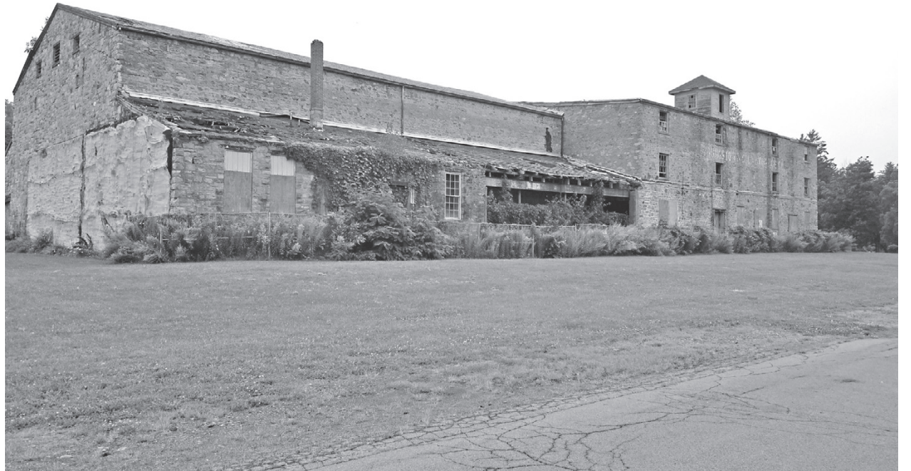
The Youngstown Cold Storage complex across from Veterans Park on Third Street.
